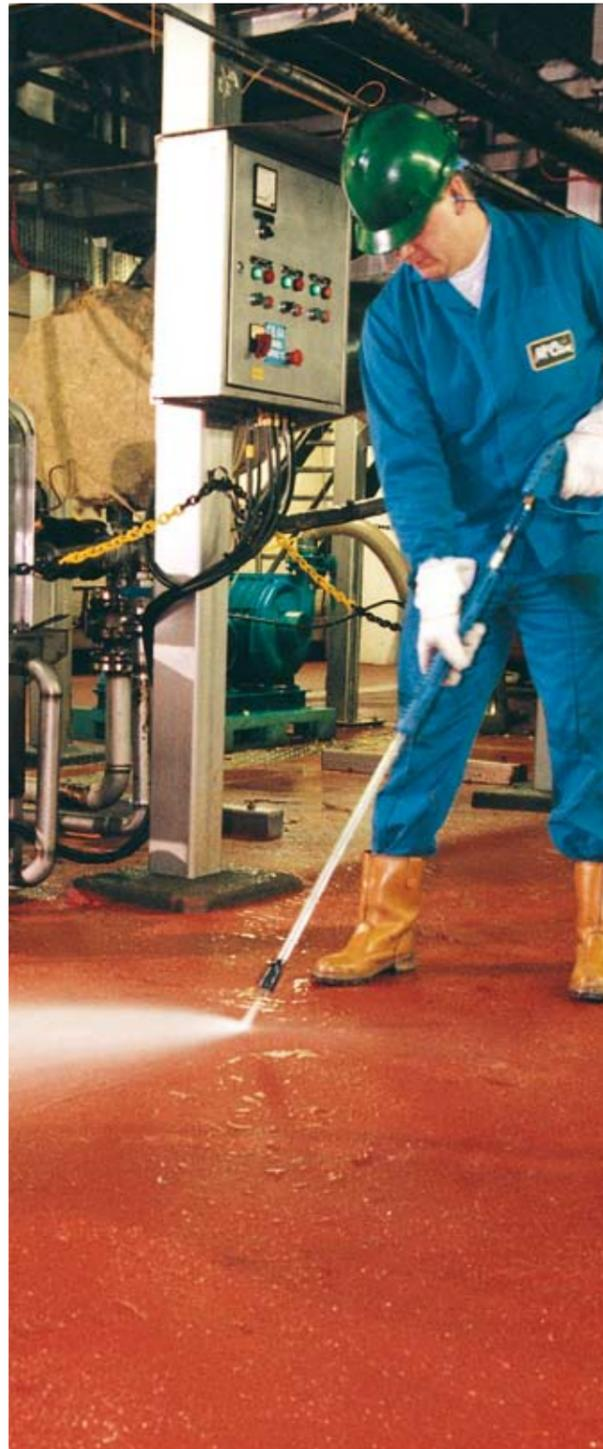
The unique UCRETE® heavy duty polyurethane resin systems do not start to soften until temperatures of 130°C are exceeded. Most other resin flooring materials soften at temperatures in the region 50°C – 60°C. Together with the high resilience of UCRETE® floors, this enables them to withstand high temperatures and extreme thermal shock conditions. UCRETE® industrial flooring is able to withstand routine and regular discharges of boiling water.
