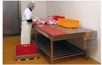
The very chemical resistant nature of UCRETE® industrial flooring means that no commercially available cleaning compounds will damage the floor when used at their normal concentrations. Puddling of cleaning solutions if allowed to evaporate to dryness may lead to deposits on the surface and 'water marks' which can be hard to remove subsequently. It follows that removal of cleaning solutions and adequate rinsing is required to maintain your floor looking its best.
